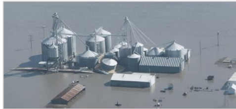
10 Grain elevator flood, Iowa USA 2019
