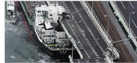
5 Infrastructure storm damage (Typhoon Jebi), Japan 2018
